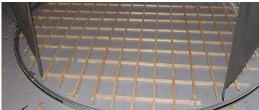
Fig. 5) Lattice structure from square timbers under the base plates
