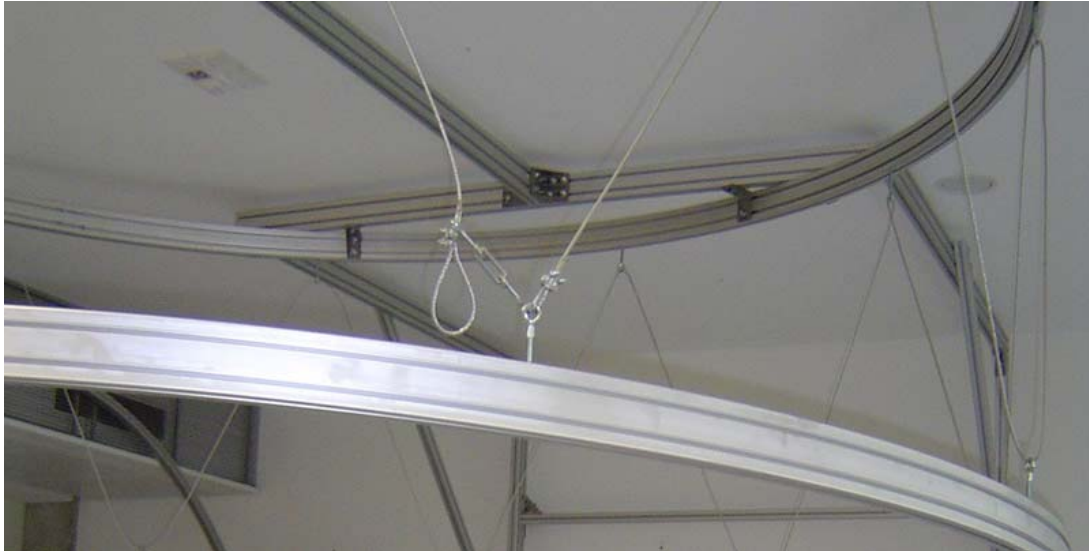
Fig. 4) Suspension of the upper cylinder ring at the carrier ring
